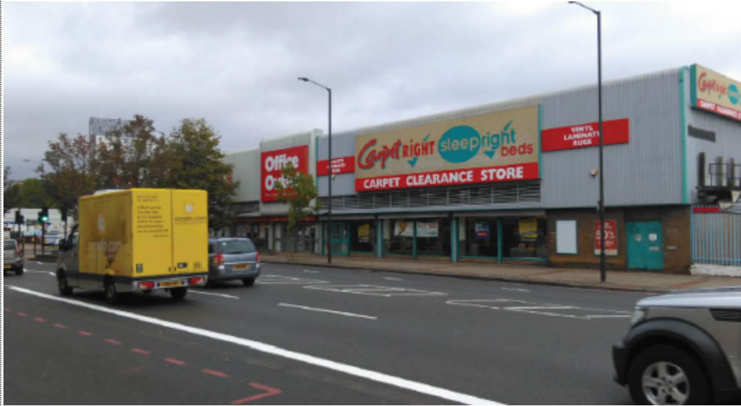
Current Site (View from Old Kent Road)
